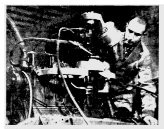
Testing a turbo or exhaust driven supercharger for automobiles he designed and built, Ray Besasie, Milwaukee automobile mechanic and inventor, says that General Motors, Inc., and the Le Roi Co. report the supercharger increases compression to six and one-half pounds above atmospheric pressure, while limiting the back pressure from the exhaust to two and one-half pounds.
